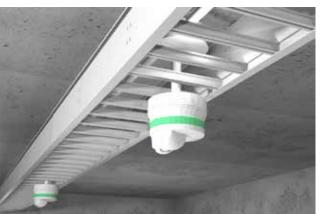
The sensor is completly obstructed by the obstacle
