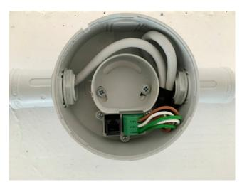
Place the wire around the inner part of the base to avoid damage to the isolation of the cable.
