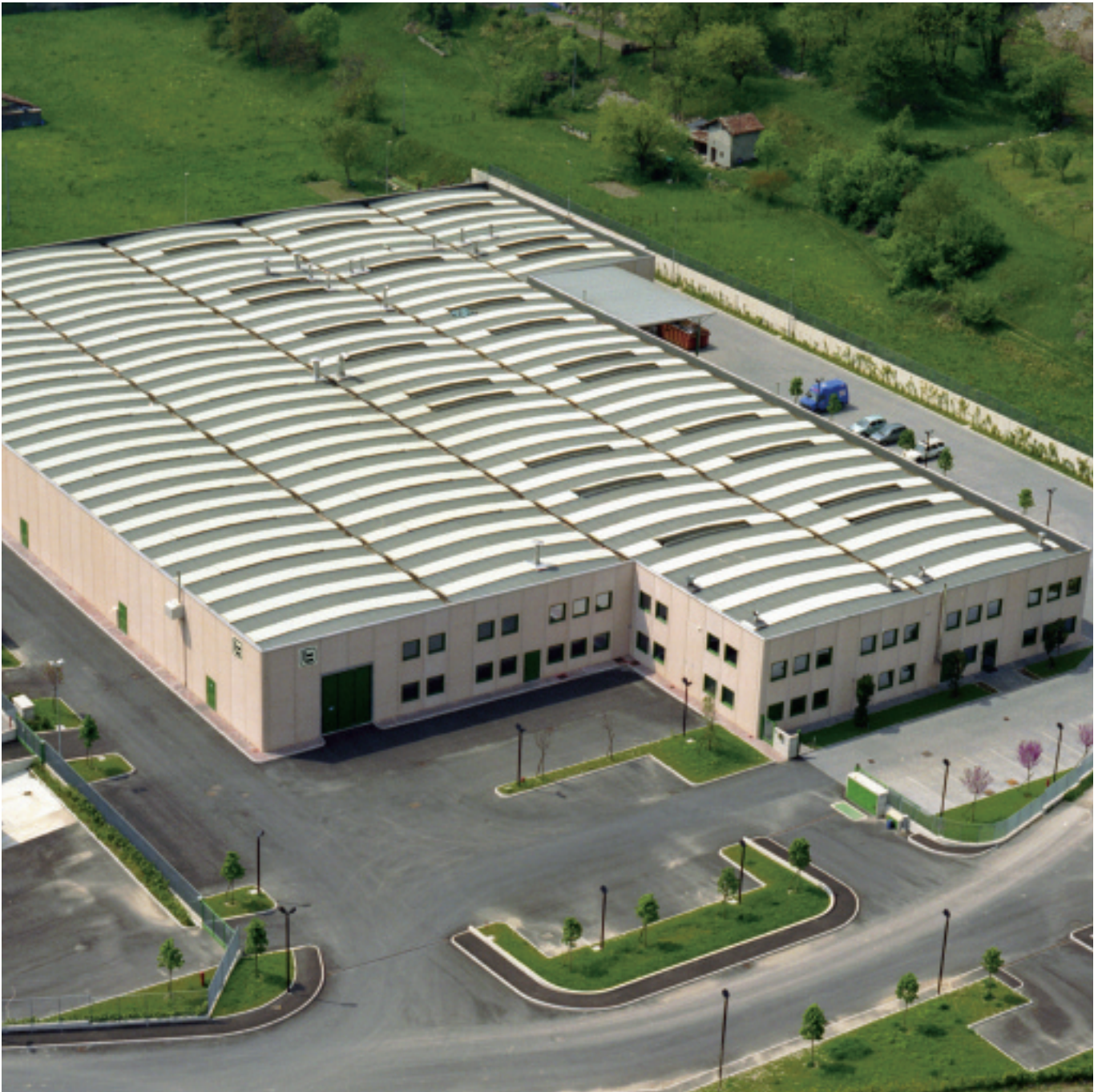
Asso, aerial view of the main facility of Special Eta and the manufacturing site of stainless steel enclosures.
